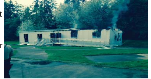
Highland Park Middle School portable fire 2014
